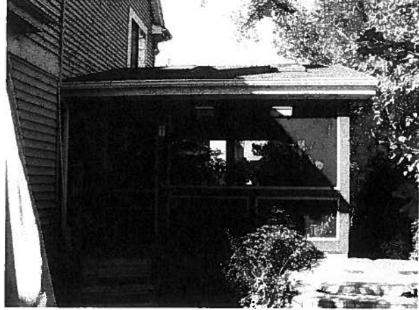
Subject screened porch addition (southern porch elevation).
