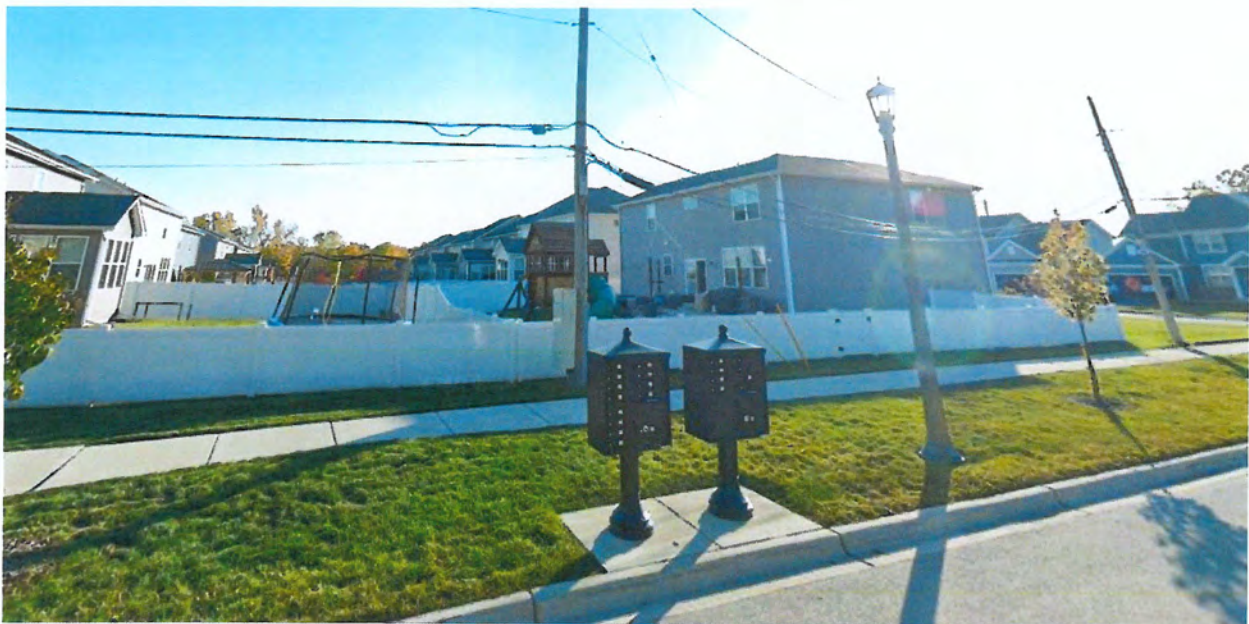
CMU at Finley Park Subdivision
