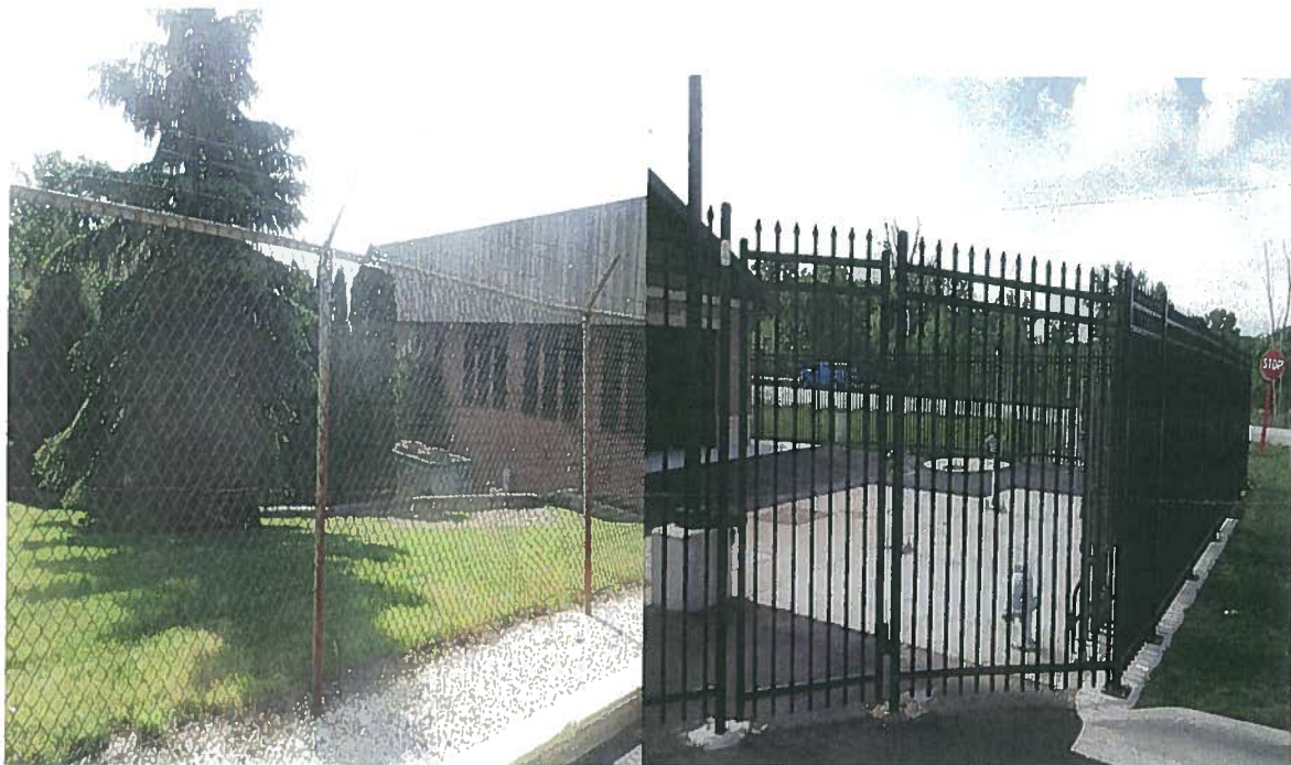
Existing 35 Year Old 6' Chain Link Fence
