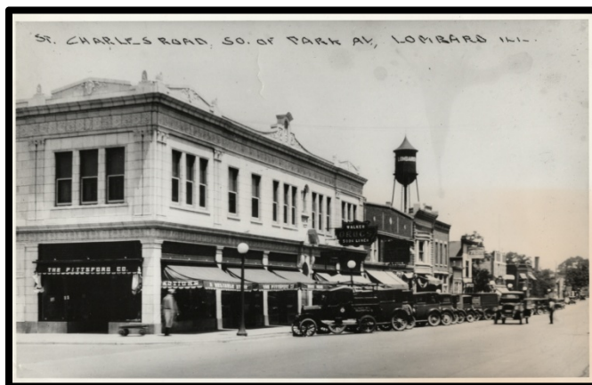
Figure 2 Historic view of original façade courtesy of Lombard Historical Society
