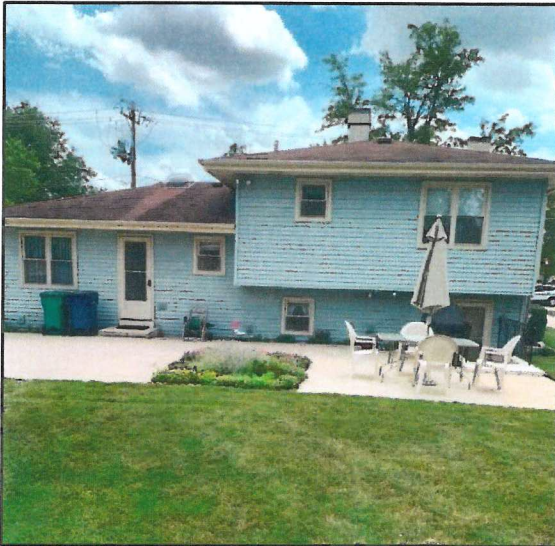
Figure 2. Rear (north) elevation of subject property.
