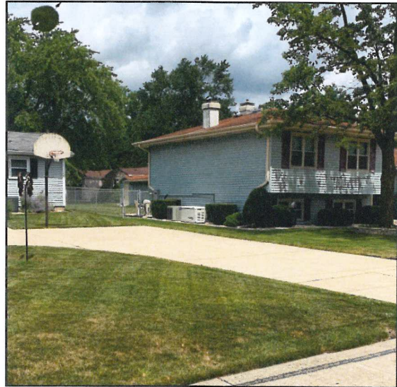
Figure 3. Side (west) elevation.
