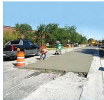
The Village's installation of Ultra-Thin Whitetopping, which is not typically used in urban areas, extends the life of the existing pavement and has earned the Village recognition from the concrete industry and local municipalities. This process extends the life of the existing pavement by up to 10 to 15 years but costs considerably less than full reconstruction.
