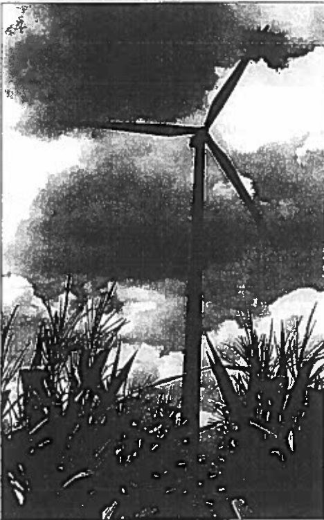
Clean Harvest: Waverly Light & Power in Iowa has installed wind turbines on land leased from local farmers, creating clean electricity for the city and additional income for farmers.
