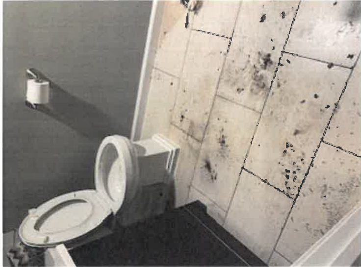
Bathroom 3 before demo
