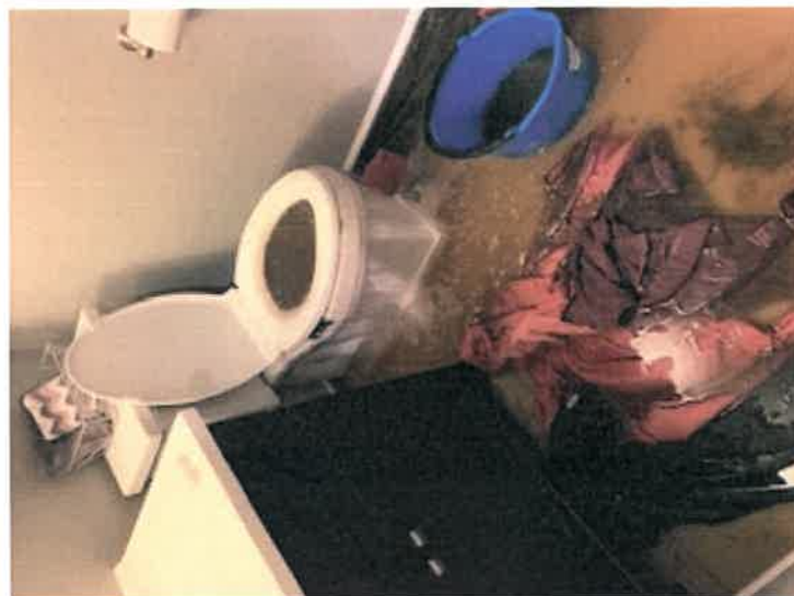
Bathroom 2 during flood
