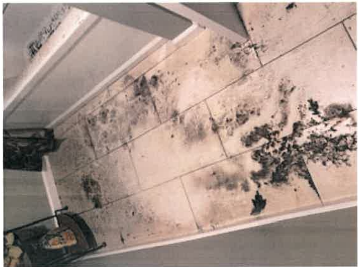
Bathroom 2 before demo
