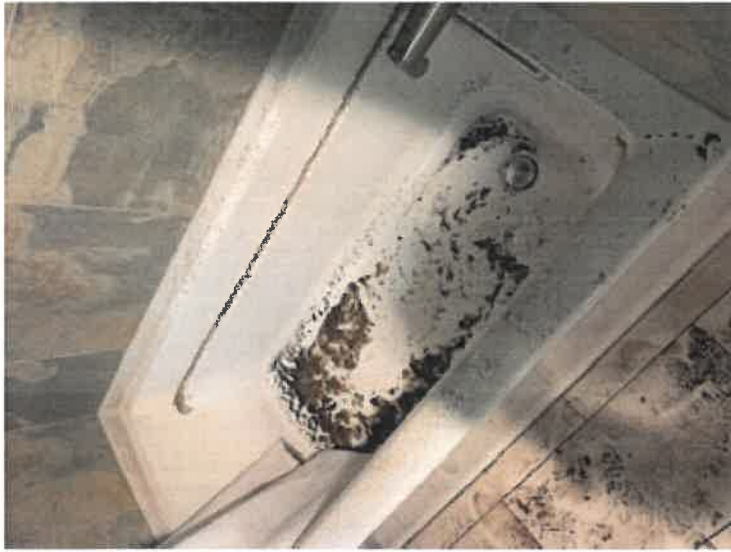
Bathroom 1 before demo
