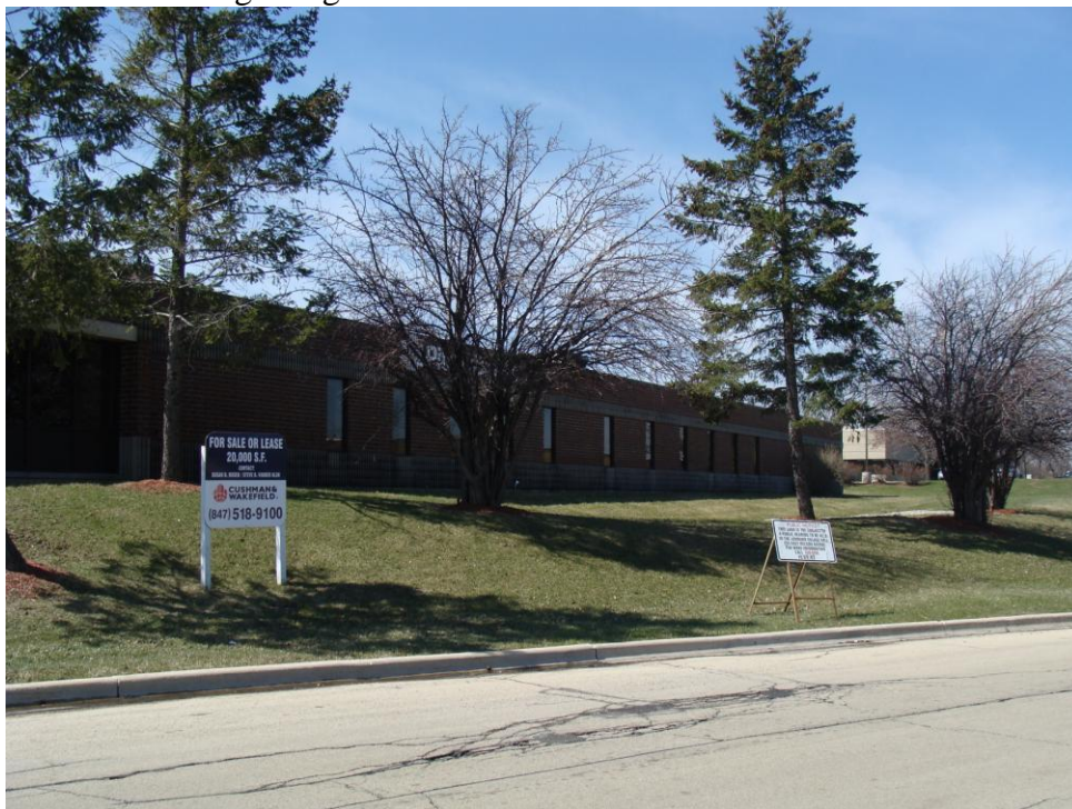
Photo 4: Front of the building along Eisenhower Lane
