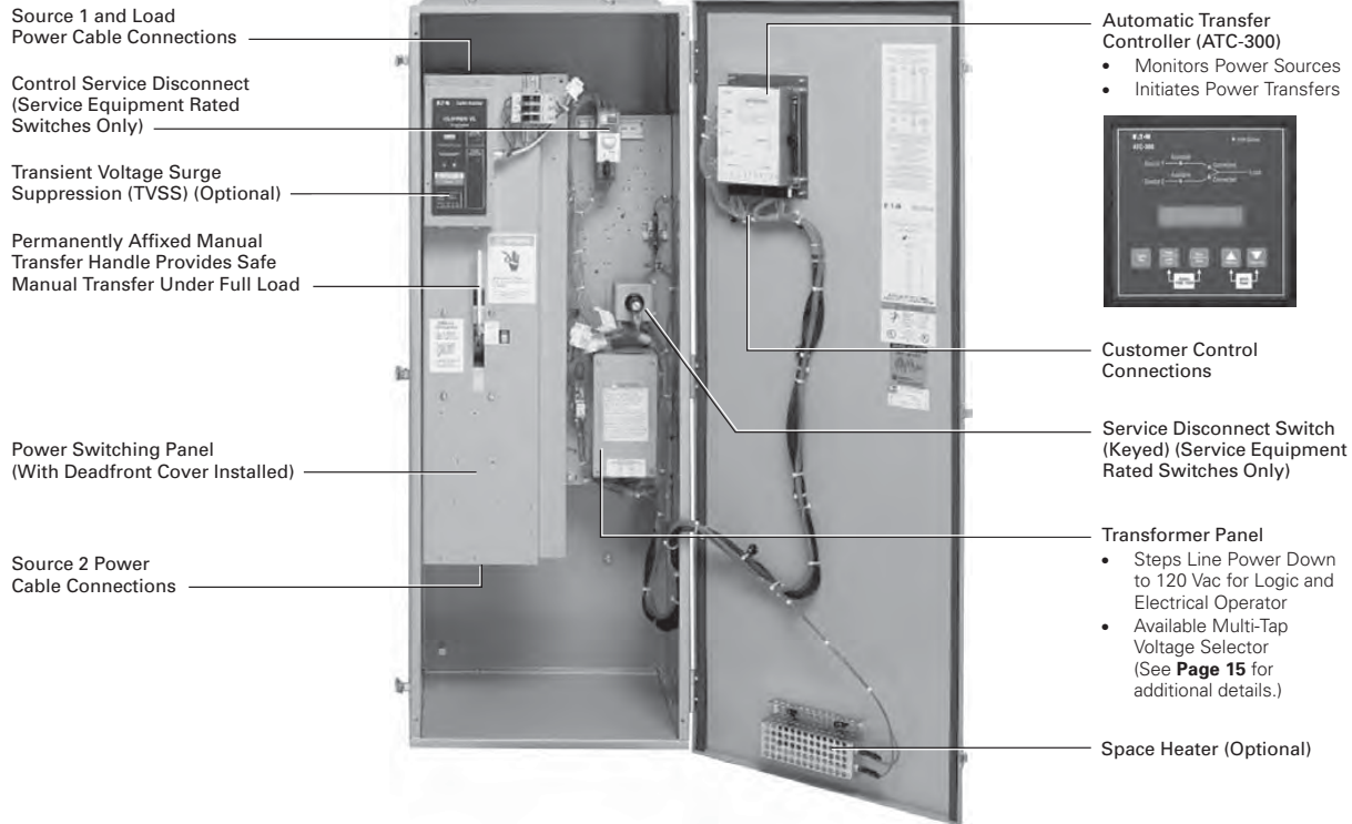
Basic Components of Automatic Transfer Switches
