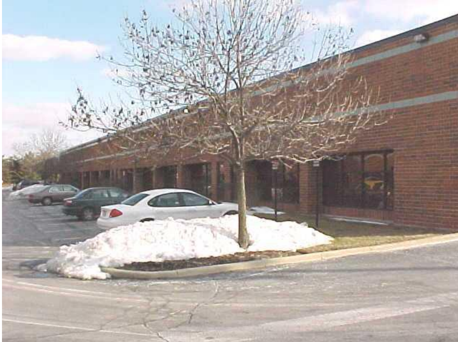
Photo 1: Northwest corner of property looking east
