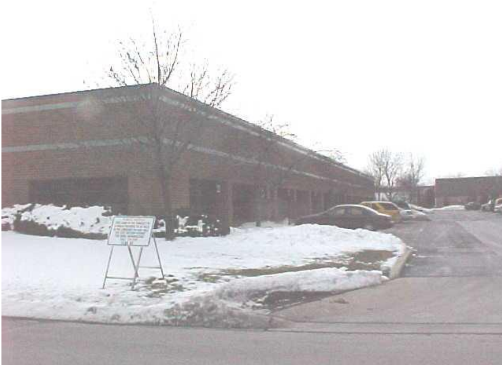
Photo 5: Northeast corner of property looking west
