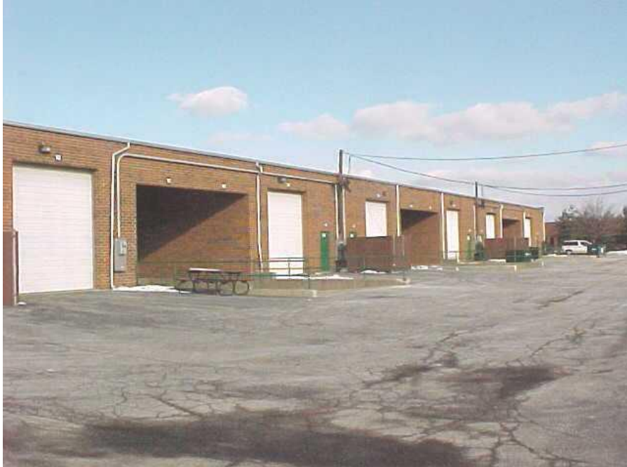
Photo 3: Southwest corner of property looking northeast
