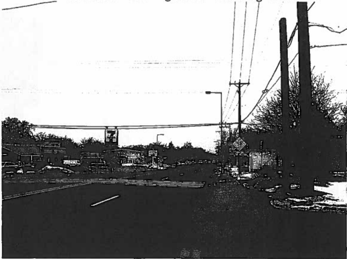
Westmore Road – looking north – Existing Condition
