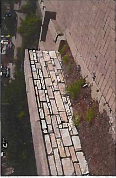
Limestone Wall with Precast Cap
