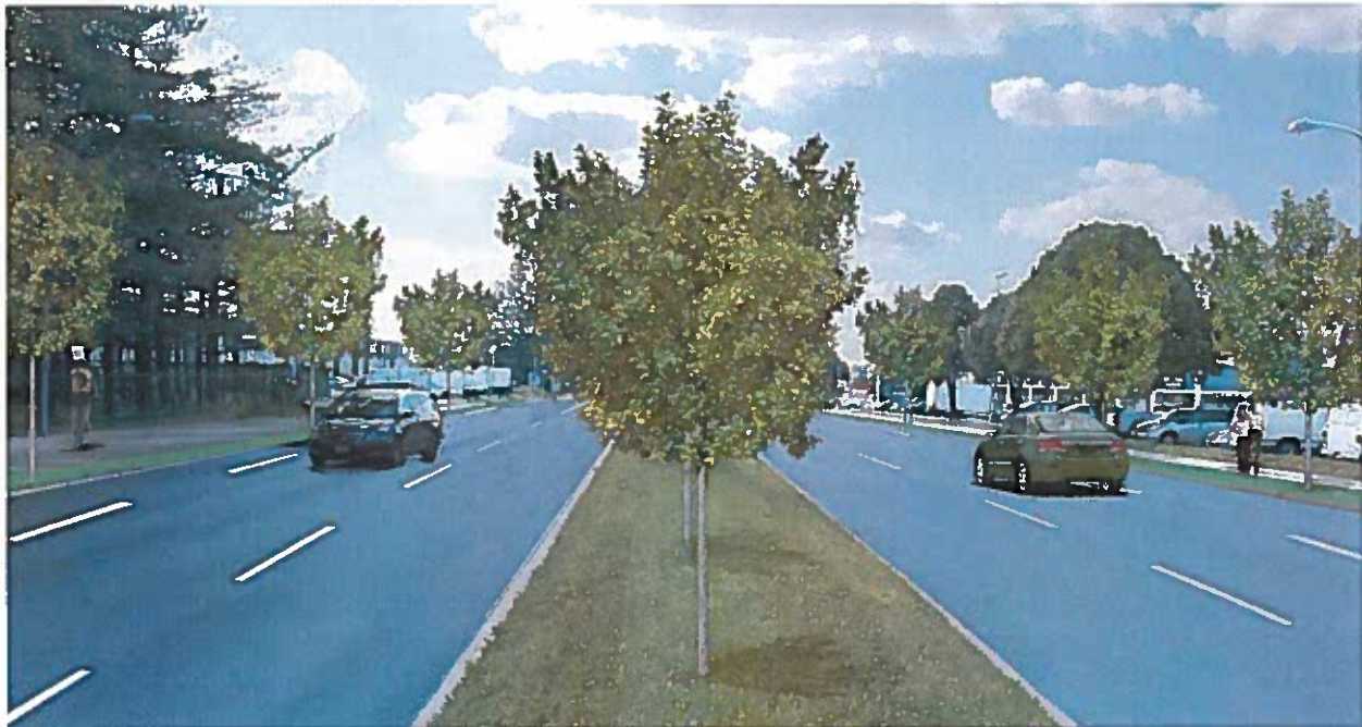
Example 1: Modifications include widening a shared pedestrian and bicycle path, widening the sidewalk, adding landscaped buffers, and narrowing and landscaping the median.
