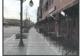
is also proposed to remain. The brick pavers beside the concrete walking surface will follow the Downtown Revitalization Guide color palette, and the pavers will be inlaid into the concrete surface to minimize future settlement of the pavers. The paver area will generally extend from the edge of the tree vaults to the curb line, as depicted in the above example image.
