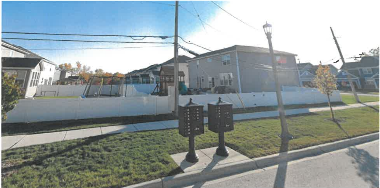
CMU at Finley Park Subdivision
