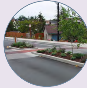
Median Refuge Island
