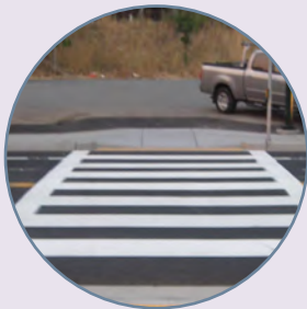
Crossing Marking Improvements
