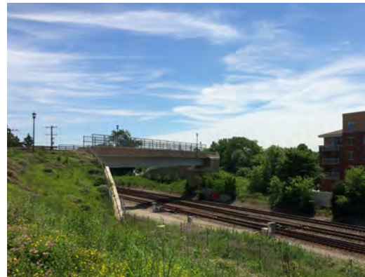
Great Western Trail Overpass at Metra Train Tracks near St. Charles Road
