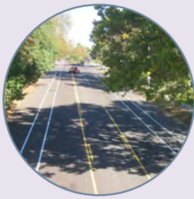
Right-of-Way Reallocation ("Road Diet")
