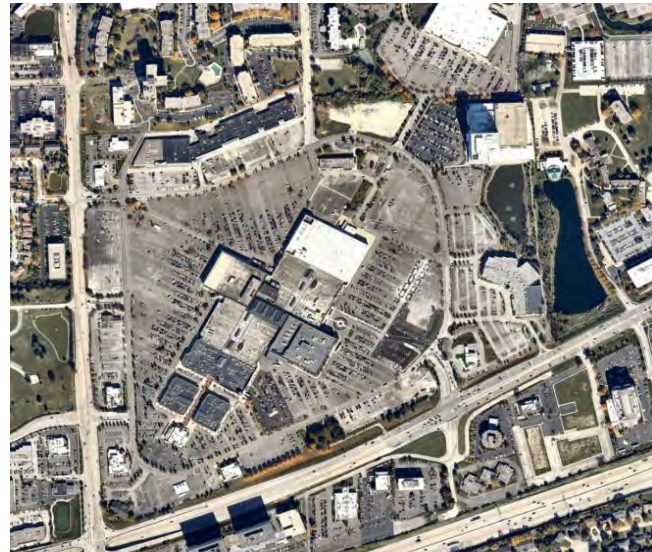
Existing conditions (Image source: nearmap.com)
