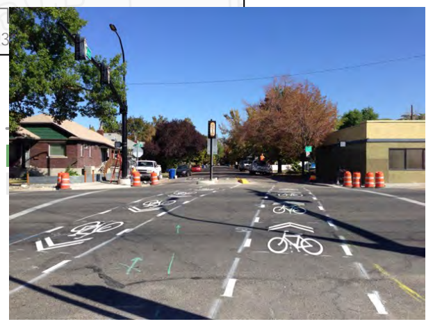
Bike lanes should include intersection markings that depict bicyclists' travel path through crossings. Such features allow drivers to anticipate bicyclists in intersections.
