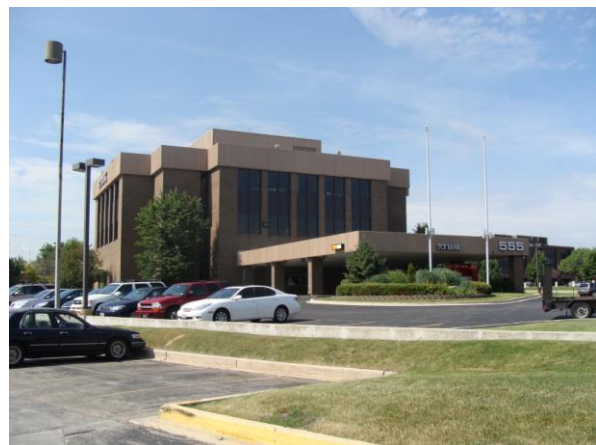
Existing office building with bank and drive-through at 555 E. Butterfield Rd.
