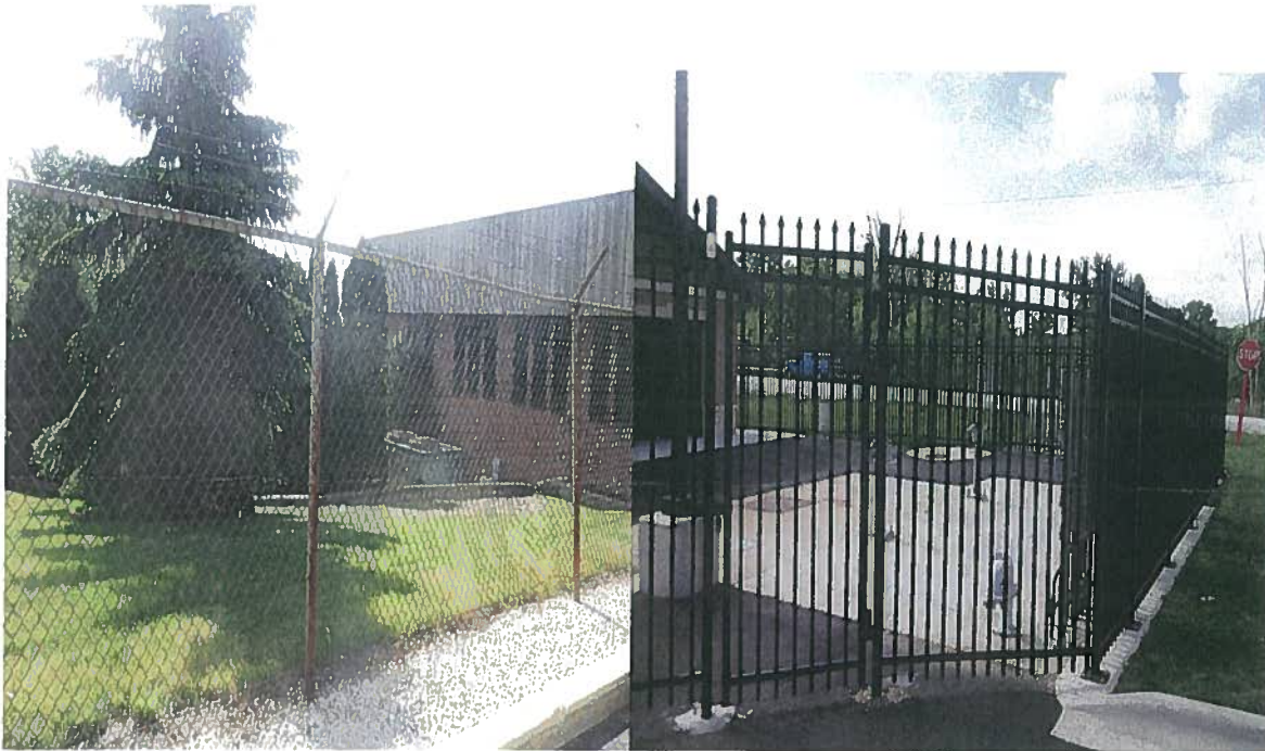
Existing 35 Year Old 6' Chain Link Fence
