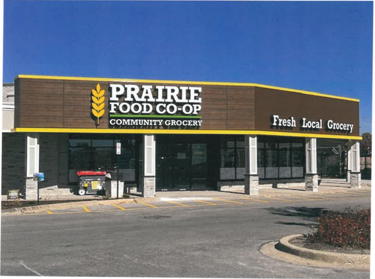
Photograph of Erected Channel Letter Wall Signage
