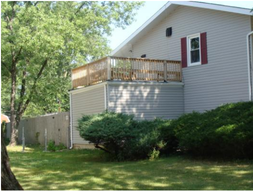
(A diagonal view of the addition and deck)
