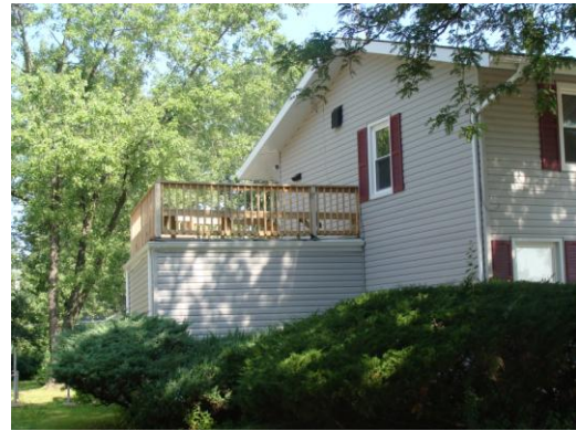
(A front view of the addition and deck)
