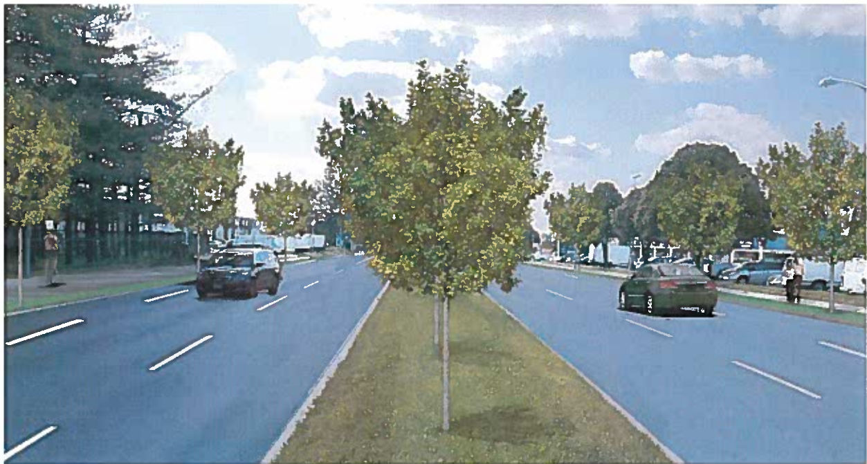
Example 1: Modifications include widening a shared pedestrian and bicycle path, widening the sidewalk, adding landscaped buffers, and narrowing and landscaping the median.
