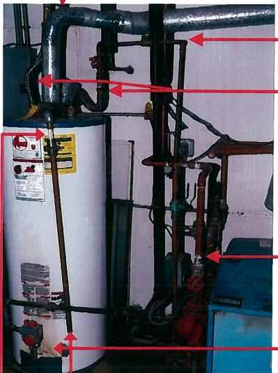
Backflow protection missing from boiler section 890.1130
