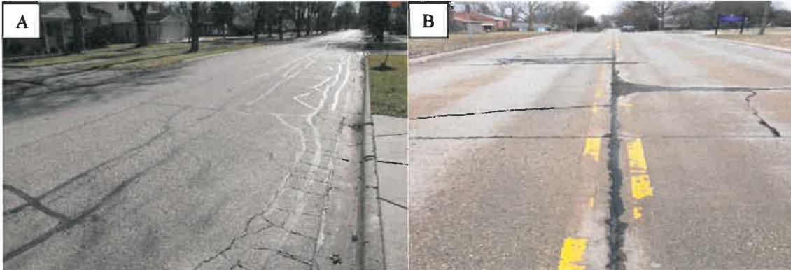
Figure 9: (a) Edson Ave between Wilson Rd and Central Ave with a 52 PCI (b) Wilson Rd between Hammerschmidt Ave and Stewart Ave with a 52 PCI
