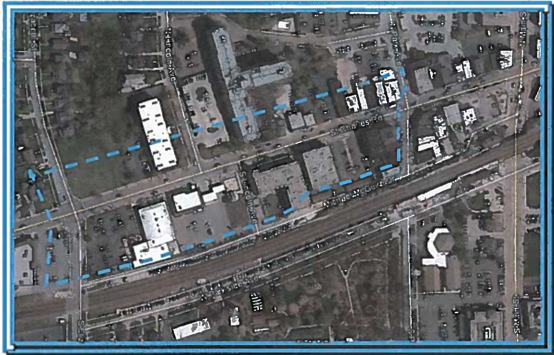
AERIAL VIEW OF STUDY AREA
