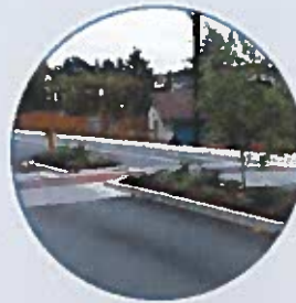
Median Refuge Island
