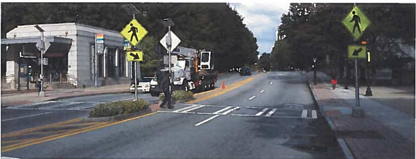
An example of a Rectangular Rapid Flash Beacon (RRFB) and pedestrian refuge island.
