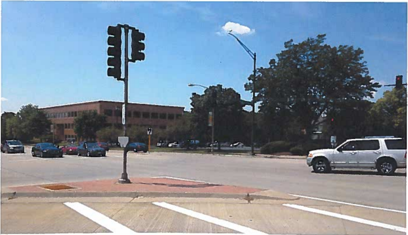
Sidepaths in southern Lombard will use a familiar type of infrastructure treatment to enable bicycle and pedestrian access to popular destinations, such as Yorktown Mall.
