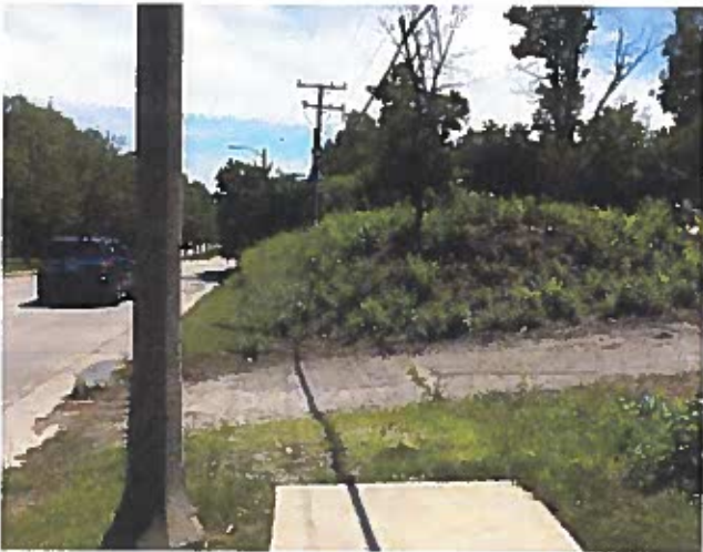
Finley Road sidepath end
