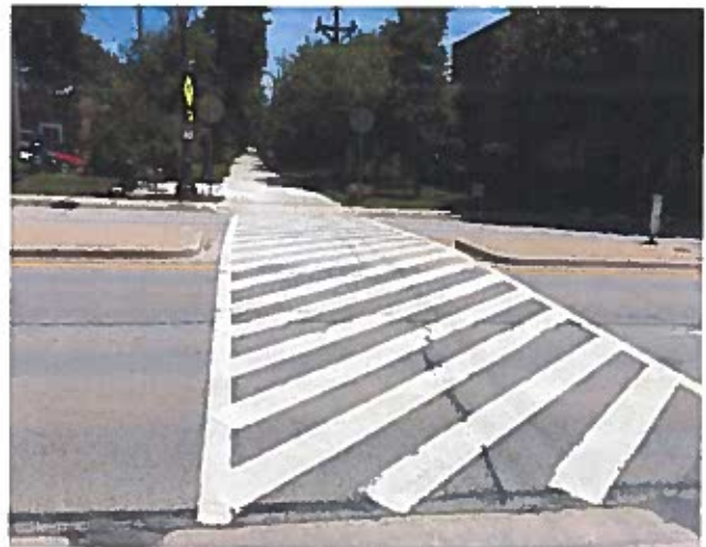
The intersection of Main Street and the Illinois Prairie Path was retrofitted with a pedestrian refuge island, yet the four travel lanes may intimidate trail users.
