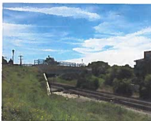
Great Western Trail Overpass at Metra Train Tracks near St. Charles Road
