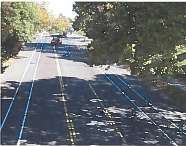
Broadway, a street in St. Louis, was restriped to include bike lanes and a center turn lane. Village officials in Lombard can undertake such projects within a street's planned resurfacing schedule.
