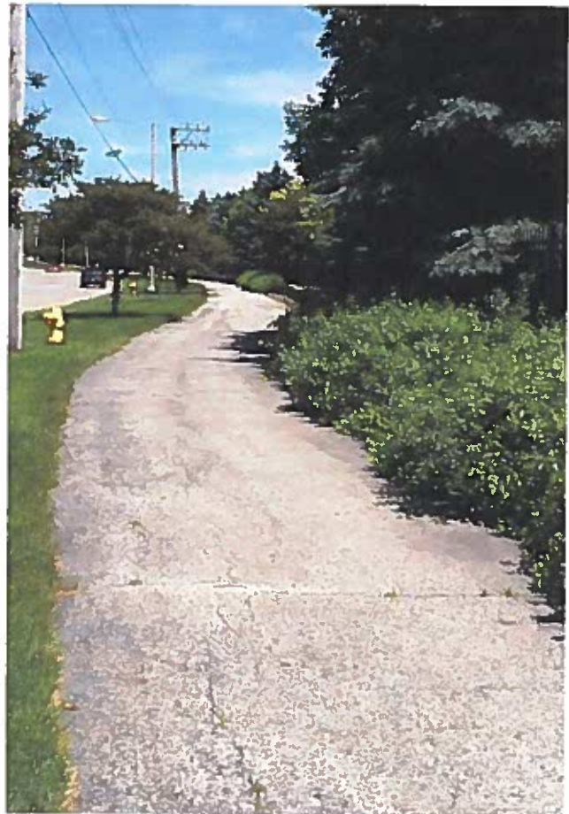
22nd Street and Finley Road sidepath
