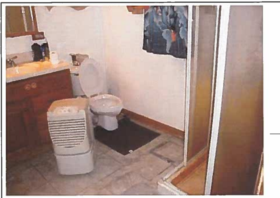
Bathroom in Basement
