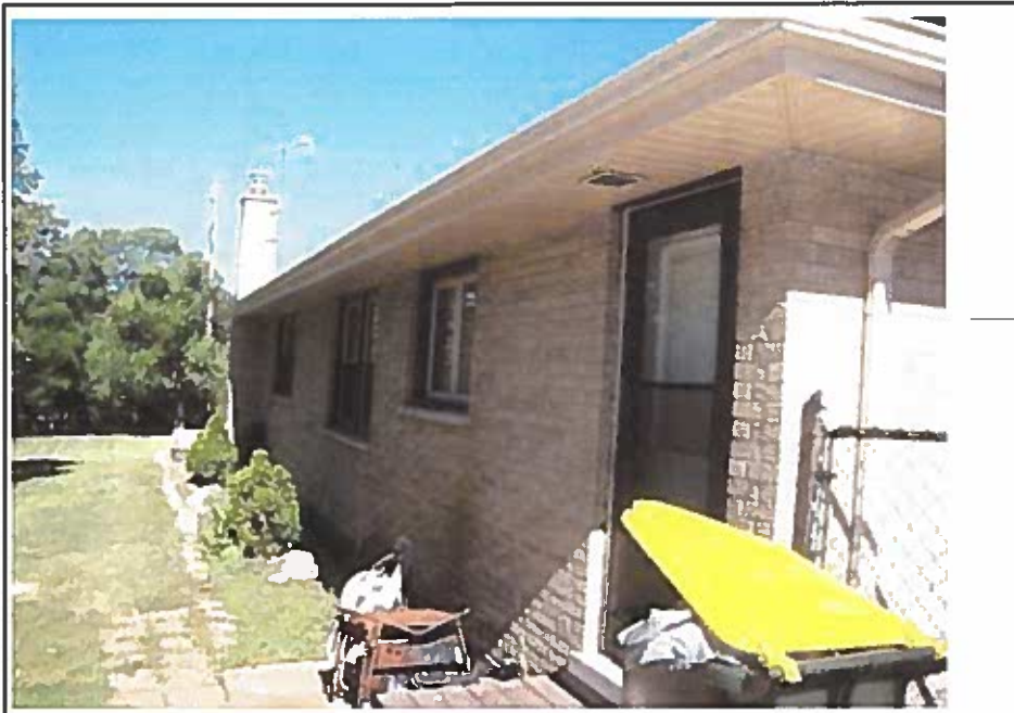
REAR OF SUBJECT PROPERTY
