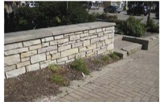
Limestone Wall with Precast Cap
