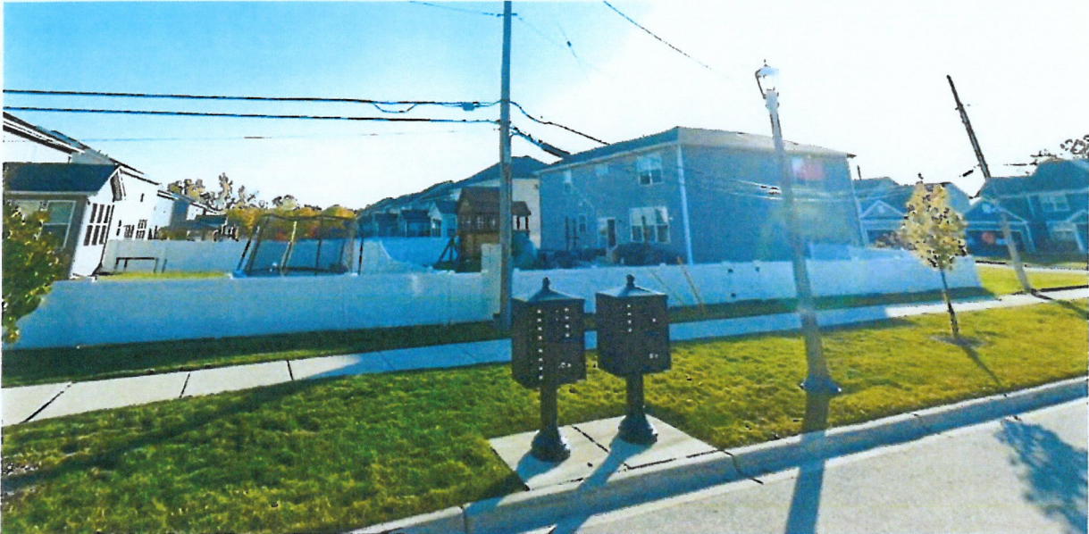
CMU at Finley Park Subdivision
