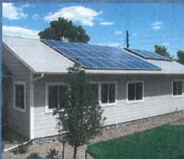
← Residential Application (5' allowable pitch accommodates flat roofs)
