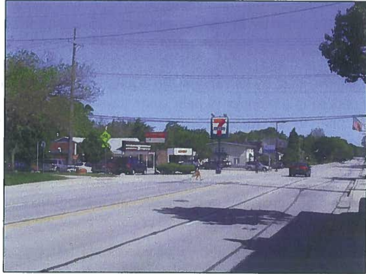
A view of Westmore-Meyers intersecting the Illinois Prairie Path.
