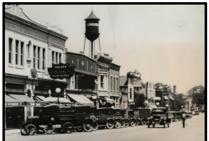
Figure 4 Historic view before CMU façade courtesy of Lombard Historical Society
