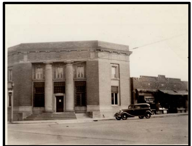
Figure 3 Historic view showing building at right, courtesy of Lombard Historical Society
