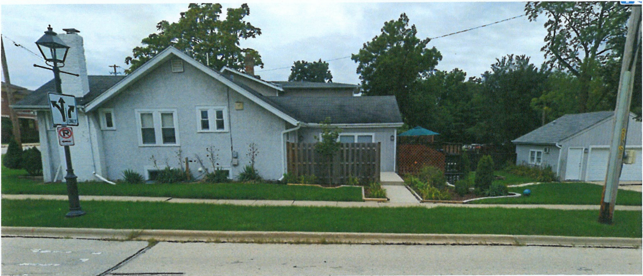
Subject property viewed from corner yard (Elizabeth Street)
