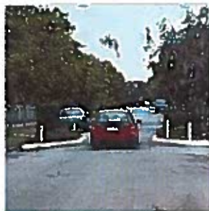
Howard County, MD – With one-lane chokers, vehicles on one side yield to vehicles from the other side until the queue is cleared, just as on one-lane bridges.
