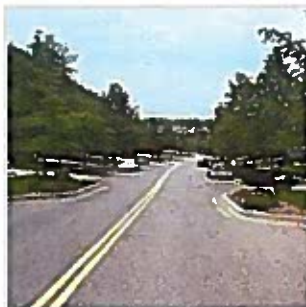
Montgomery County, MD – This choker uses slightly offset curb extensions to accommodate the residential driveways.
